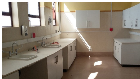
Figure 15. Renovated biorepository room.
