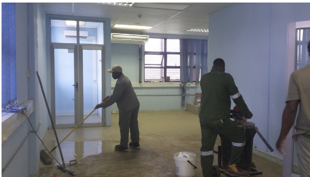
Figure 9. Renovation works Mbabane reference laboratory.
